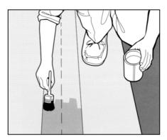
¬Apply adhesive to remaining area of wall and position sheet. Heat and stretch slightly the wall material around the corner at the same time as it is pressed firmly into the adhesive.
