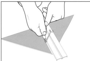
To glue the triangle-shaped piece more simply and securely, cut a groove on the back of the triangle with Tarkett Corner Knife. The depth of the groove shall be no deeper than half of the sheet thickness.
